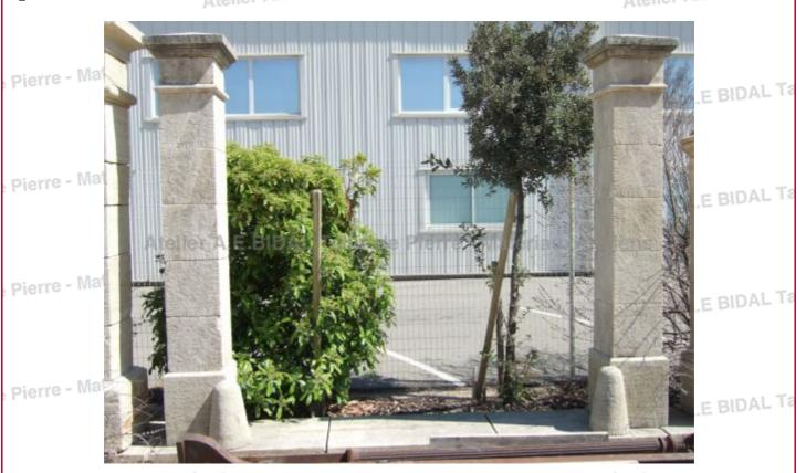
Square pillars in natural stone from France (Estaillades or Avy stone) composed of a slightly pointy capital, a central shaft made up of several elements and adorned with a large molded rim at the top, and a solid base with wheel protectors - the pair.
